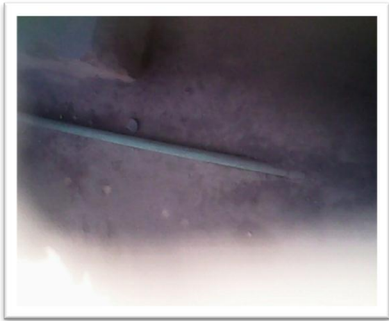
PLATE 18 PPR pipe exposed on the surface in Soweto village kayole
