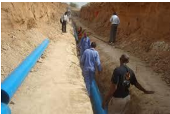
PLATE 25 Underground installation of UPVC pipes
