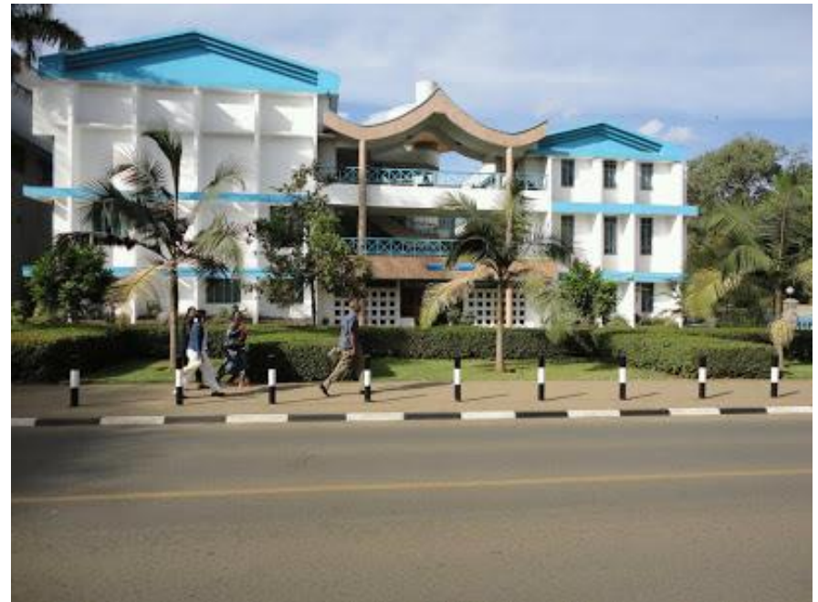
The Civil Block on Harry Thuku Road
