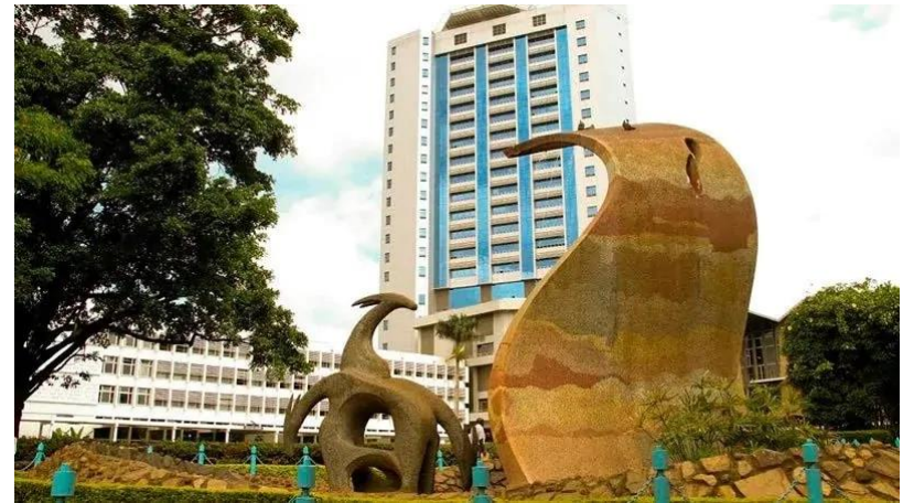
The fountain of knowledge in the foreground of the great court
