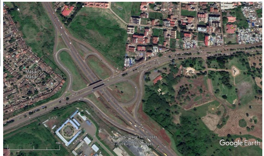
Southern Bypass Langata Road Interchange
