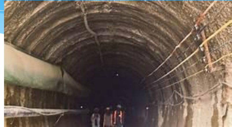
Inside the tunnel
