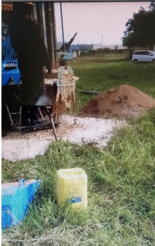
Borehole drilling in Kudho School, Kisumu
