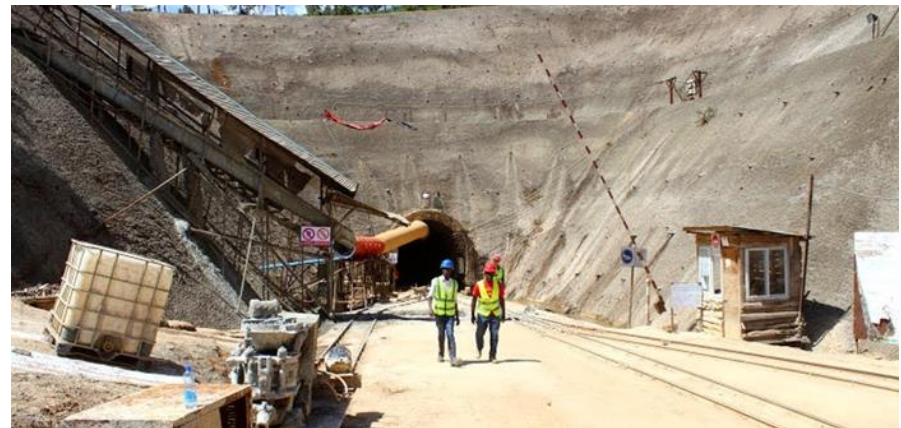
Initial tunnelling phase
