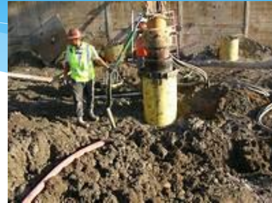
Foundation pile driving
