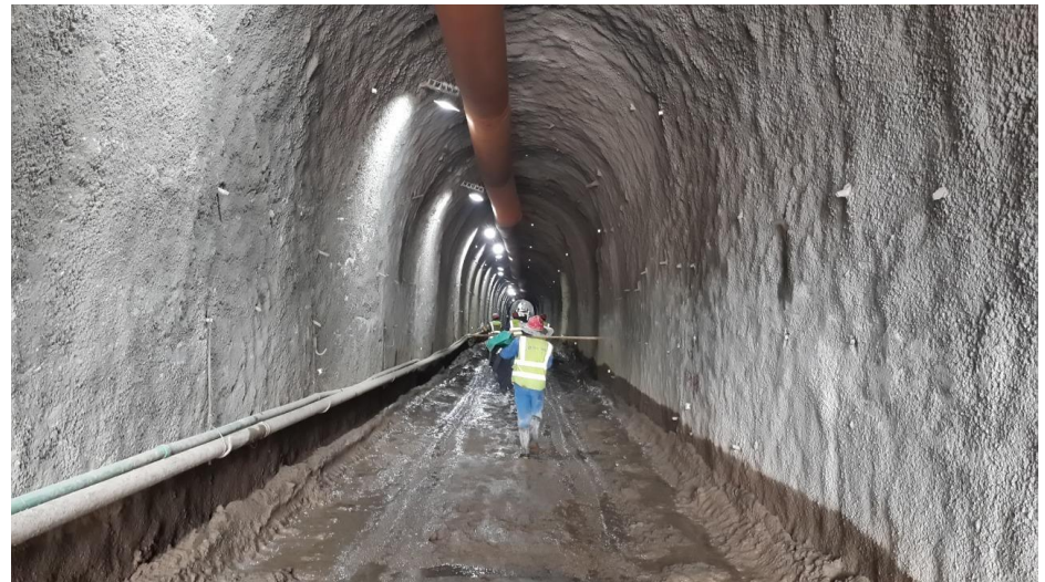
Inside a Tunnelling works in progress
