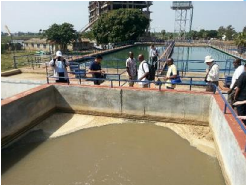
Kajulu Water Treatment Works, Kisumu
