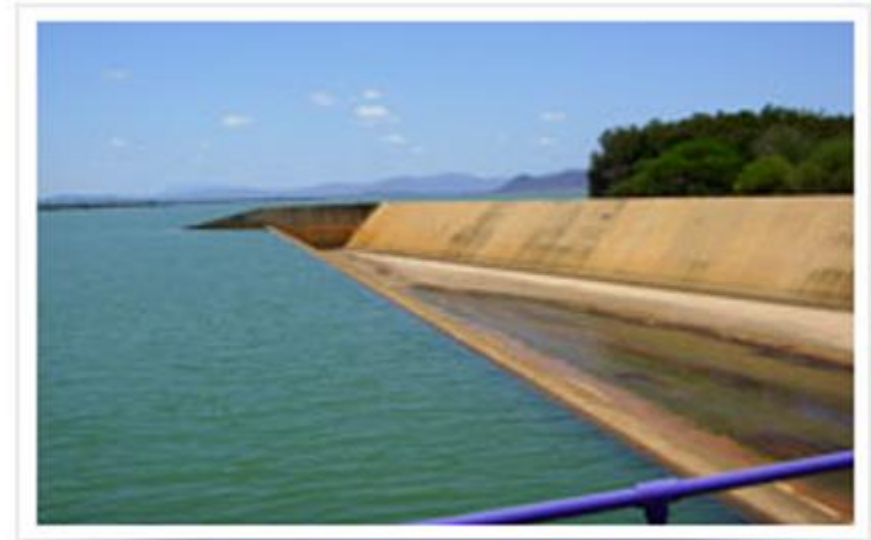
Masinga Dam Spillway
