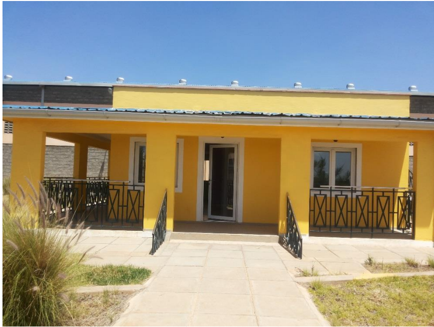
Figure 2.19 Finished EPS sample house at NHC factory
