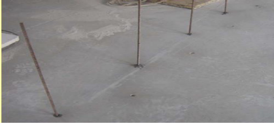
Plate 2- 14: Drilled holes in the foundation (Schnell 2014).
