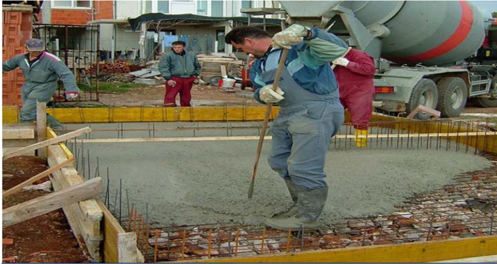
Plate 2- 12: Placement of rebars (Schnell 2014).
