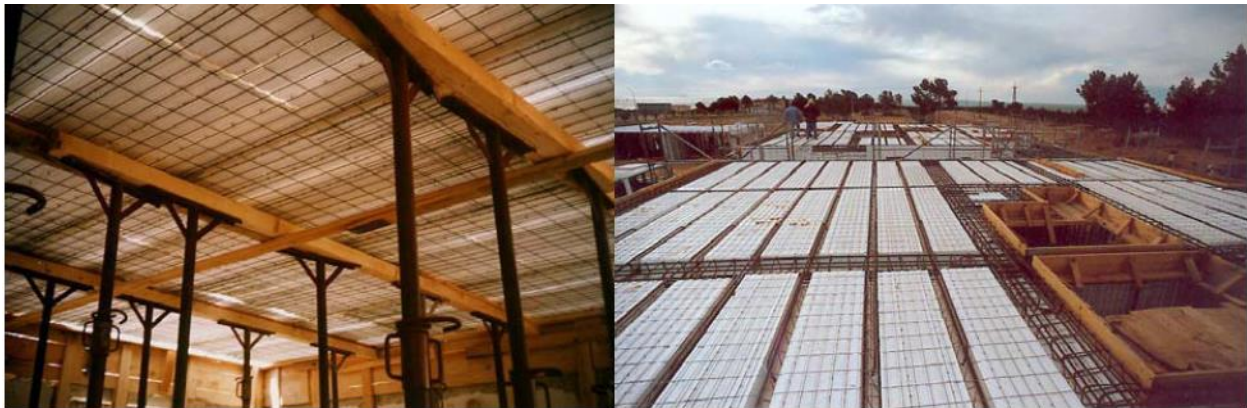
Plate 4- 8: Supporting formwork for expanded polystyrene floor panels (Emedue 2011)
