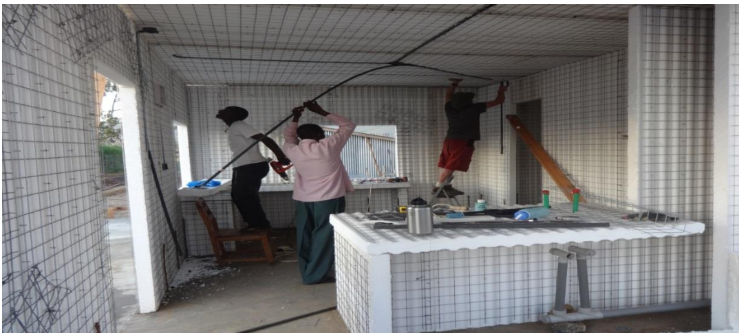
Plate 4- 9: Putting allowances for fixture and fittings (Emedue 2011)
