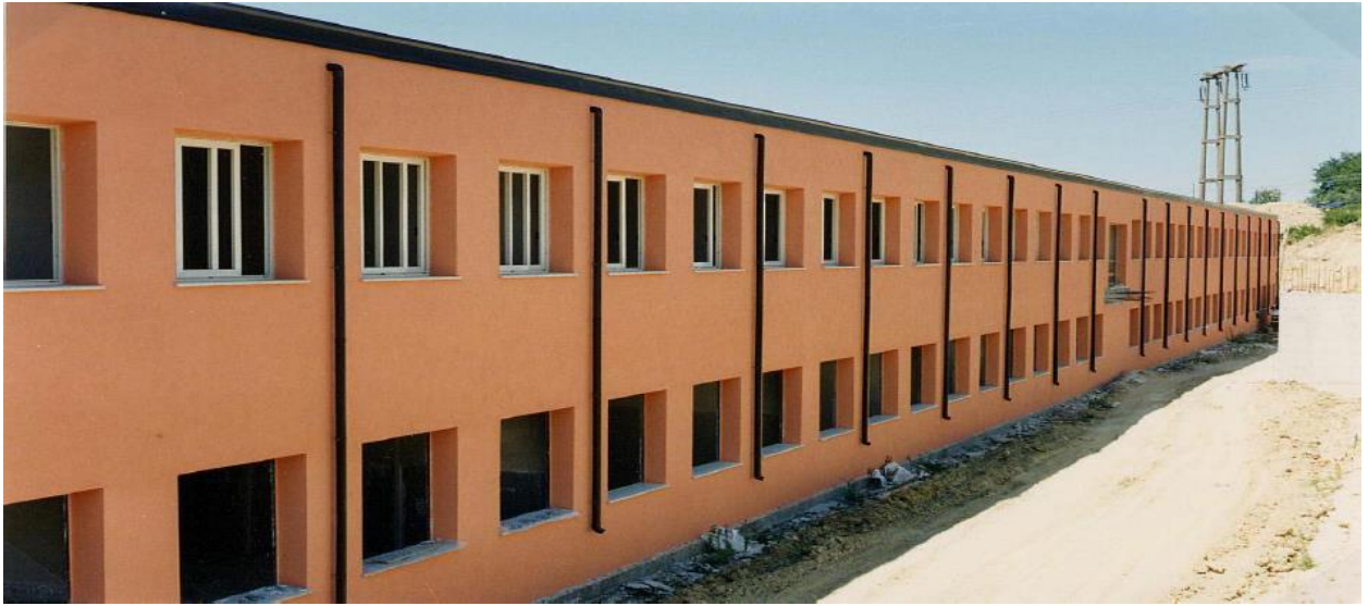
Plate 2- 2: Finished structure made of expanded polystyrene panels (Schnell 2014).
