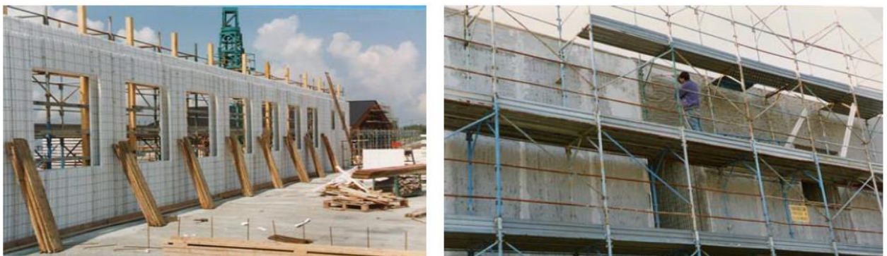
Plate 2- 1: Wall panels set up and process of spraying with shotcrete (Schnell 2014).
