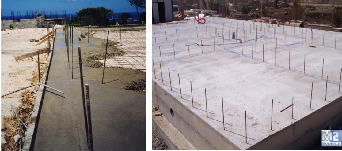
Plate 2- 11: How to anchor panels (Emedue 2011)
