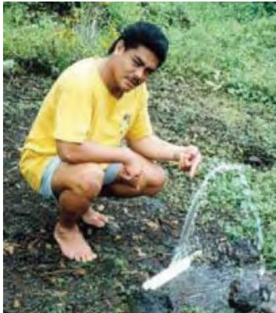
Figure 2.9: Leakage on service connections (Farley, 2008)
