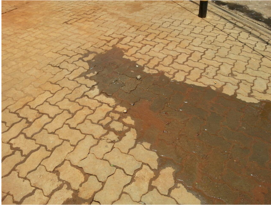
Figure A4: Leakage on service connections, Ngara Road
