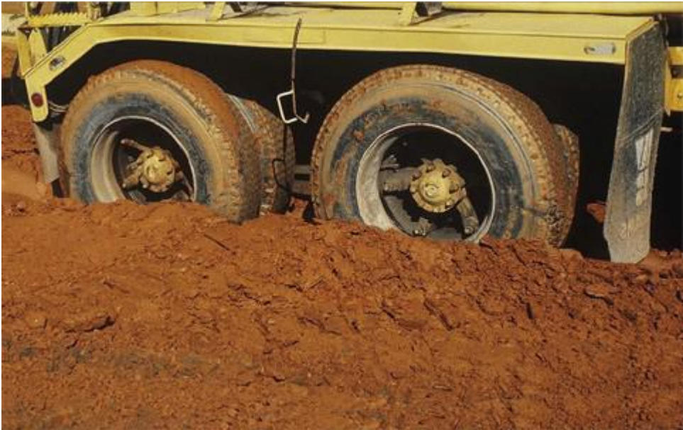
Figure 1.0 fine grained soil- difficult to compact, slow drying, and poor working platform
