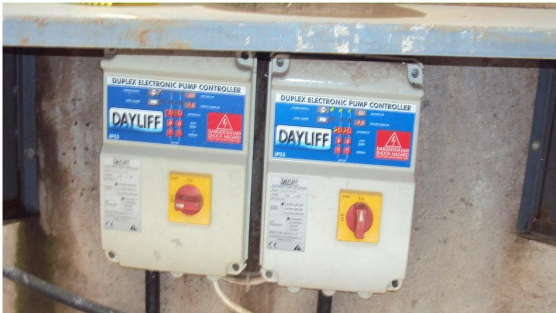
**Figure 2.5: Duplex Electronic Pump Controllers at Maasai Mall ETP**
