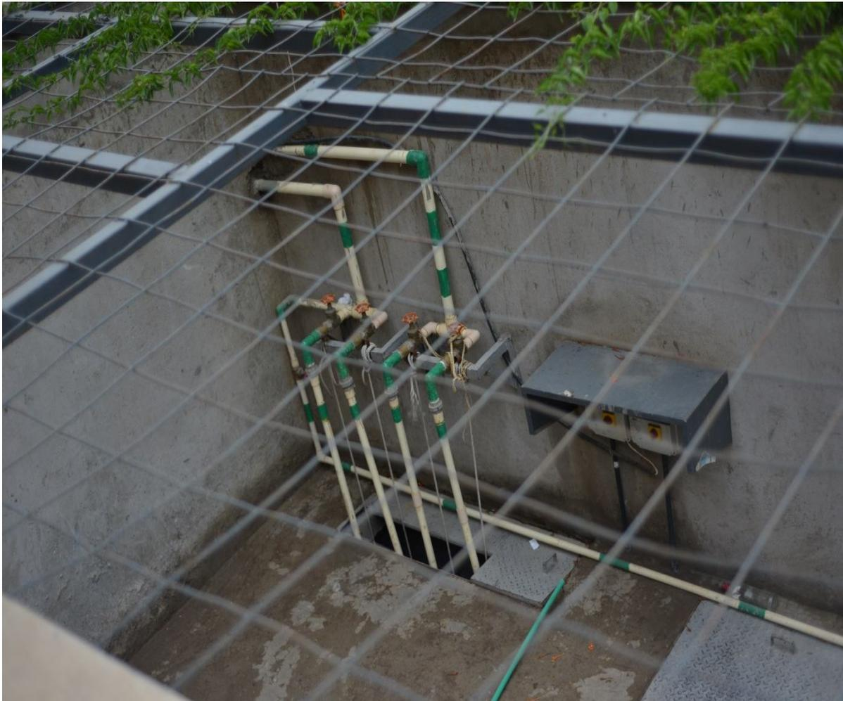
**Figure 2.6: Air-lift Sludge Return**
