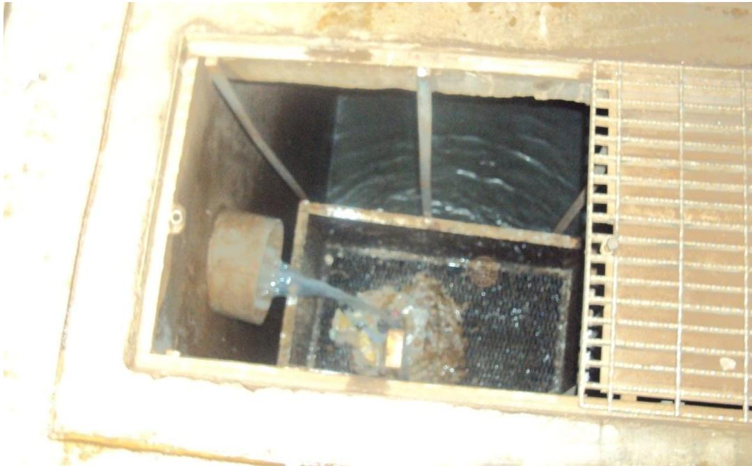
**Figure 2.3: Influent point with Trash trap and Bar Screen**
