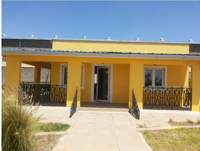
Figure 2.19 Finished EPS sample house at NHC factory
